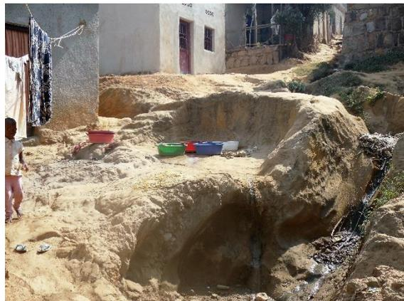
*Photo 7: Sanitation: (a) an outside pit latrine (b) a ravine draining wastes*
