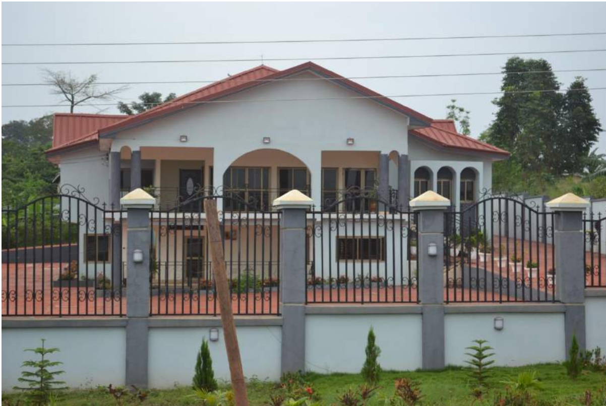
· Picture 7. Migrants invest in building structures
